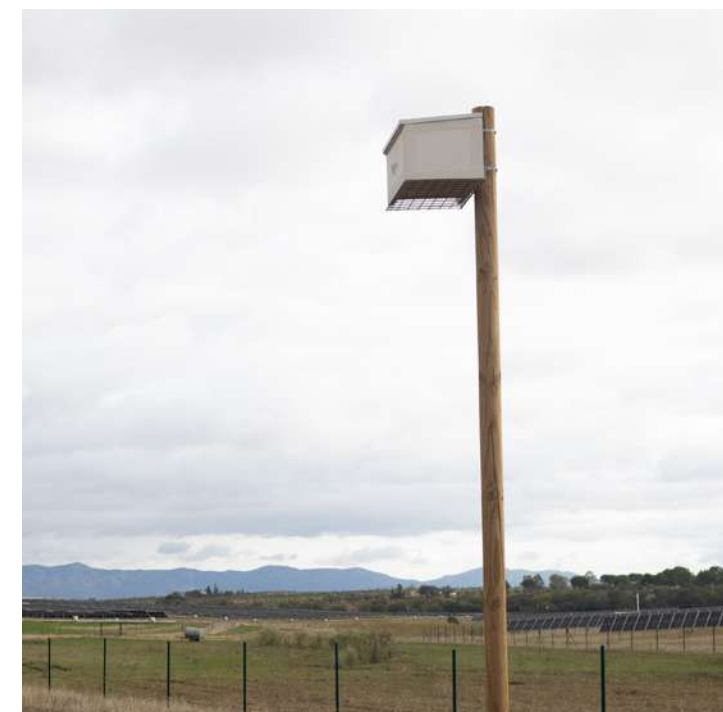
Installation of bird boxes
